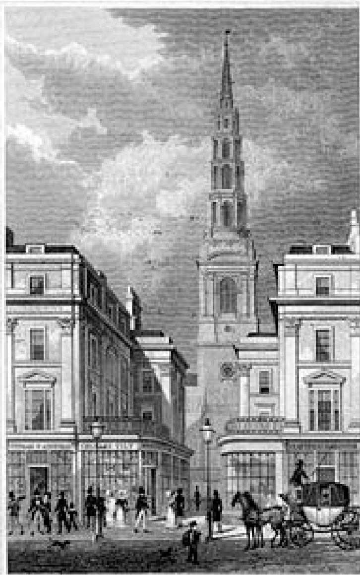
27. BRIDGE AVENUE, FIRST STREET.
